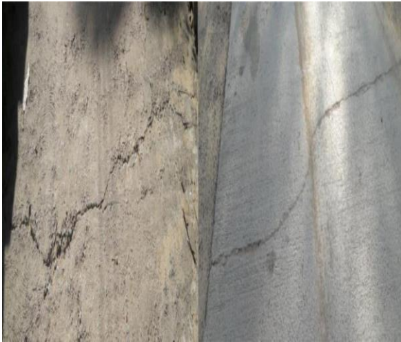
Fig. 3. Transverse Cracking
