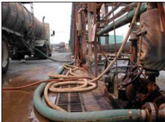
Fig. 7. View of the tankers near the leak of hydrogen sulfide [18]
