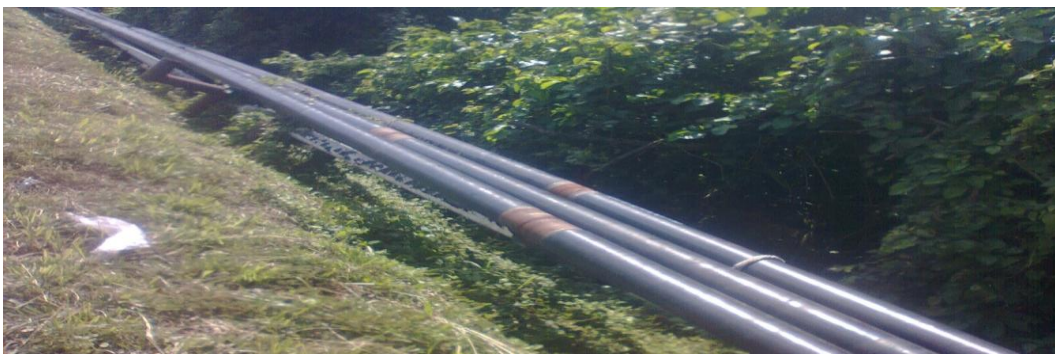
Fig. 2: pipelines running through the mangroves
